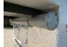
Rod / pole storage
